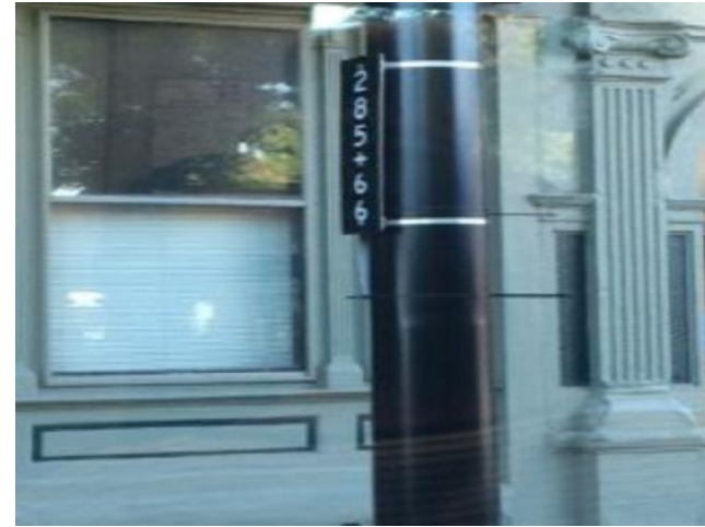
Catenary Pole Number
